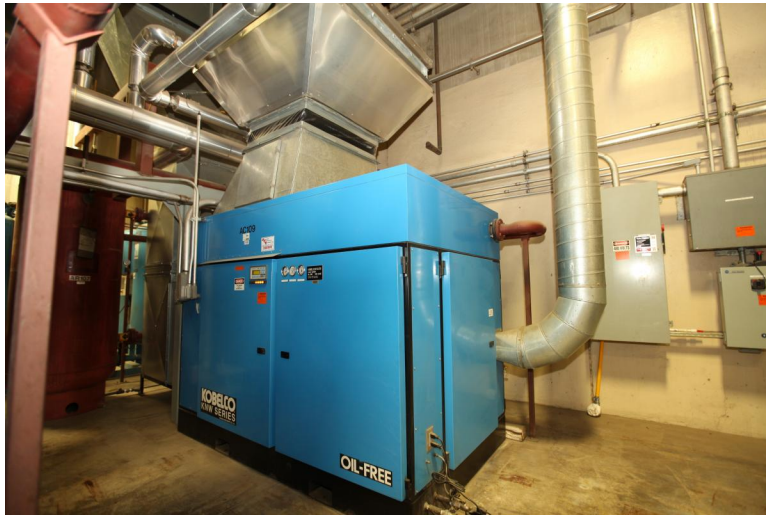
One of four Kobelco KNW series oil-free screw compressors at Nestlé’s ice cream factory. Note the air-to-water heat exchanger in the ductwork above.
